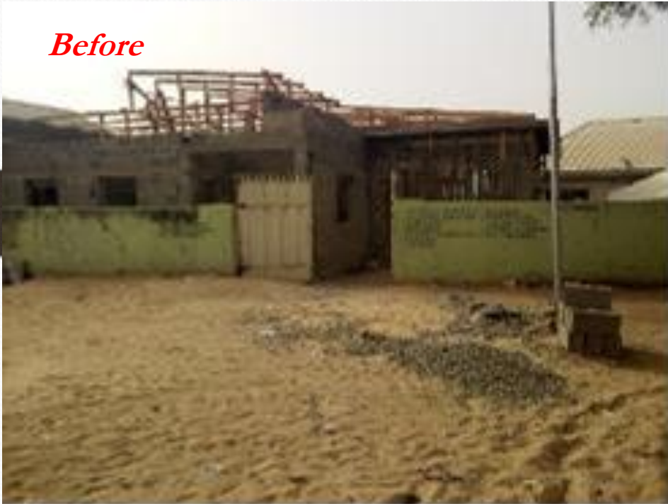
Ongoing construction in Jamputu Primary Health Centre, Yola North
